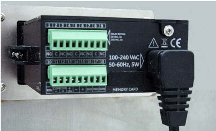
Figure 32: The AC Power Cable Installed
