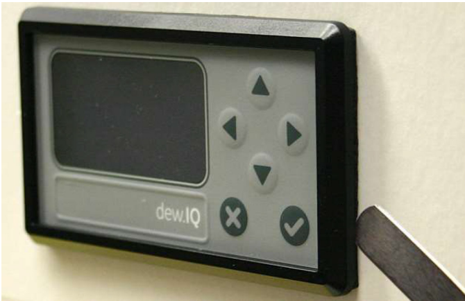
Figure 15: Checking the Gasket Compression
