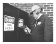
Test switchgear, transformers, etc. for arcing, tracking & corona.
