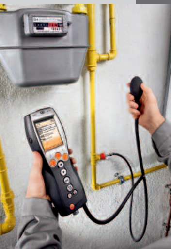
The gas pipe test
