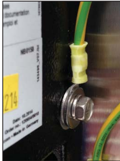
Figure 3 Earth Bolt And Nut Washer Assembly
