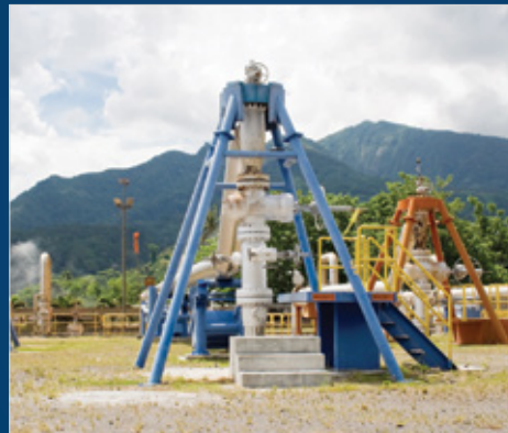
Geothermal Well Testing
