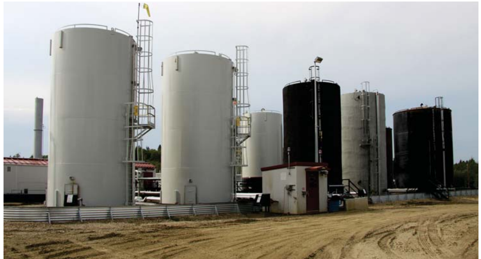
Petrobakken Energy Ltd. Crude Oil Battery, Drayton Valley, Alberta
