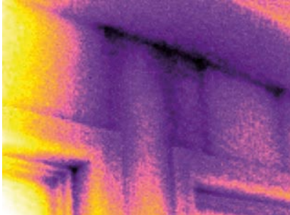
Mold remediation: Control mold by revealing undetected sources of moisture.
