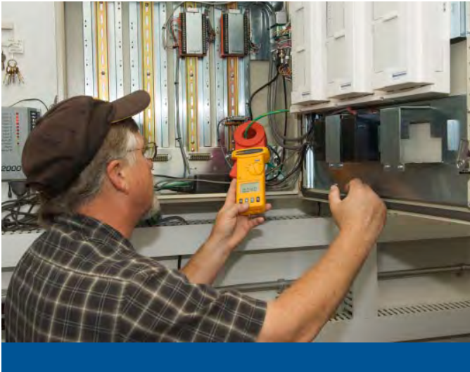
Bob Frazey uses the Fluke 1630 to check all the grounding wires around the building that all the communications come into from various points around and across the dam. These include remote sensors, video feeds, and visual and audio warning stations.
