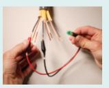
GREEN LED means wiring is properly identified.
