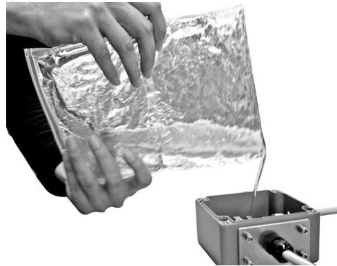
Figure 6: Pour resin into the junction box
