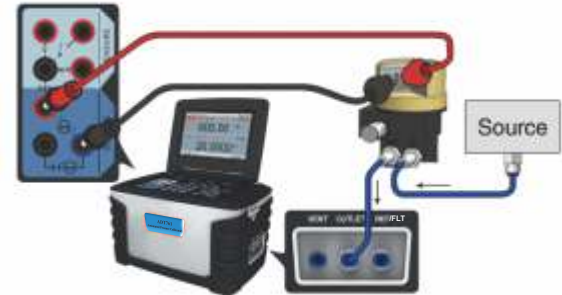
Figure 3-19 Calibrating a I/P converter
