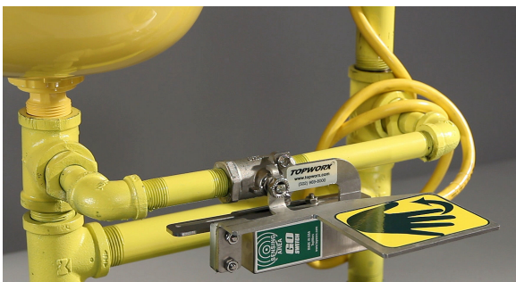
Figure 5: Eye Wash in Activated Position
