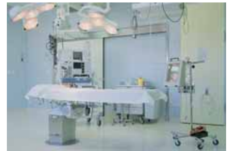
In hospitals and research laboratories, the pressure difference (negative pressure) prevents the spread of germs and dust
